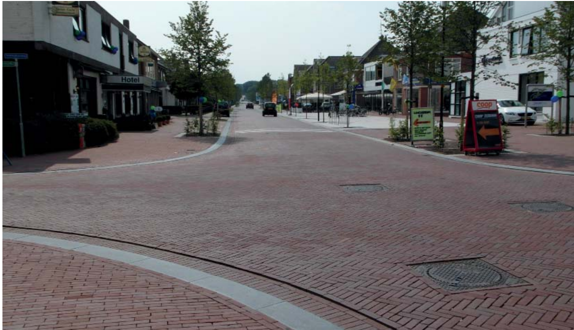
Use of the same material for car and pedestrian areas to create a level playing field (equality)
